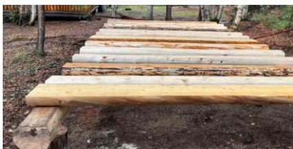
Sill logs and joists go down.
