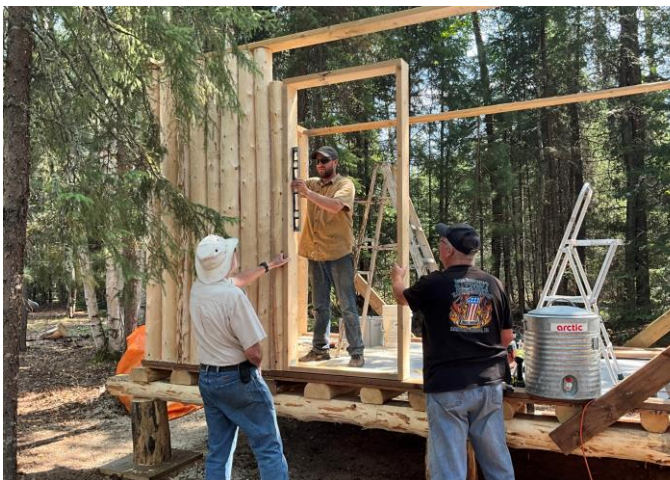
Walls starting to go up.
